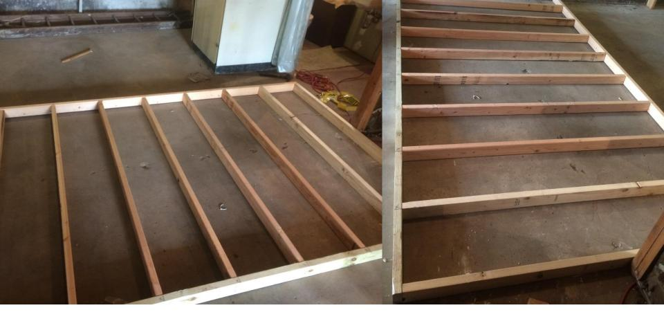
Completed wall section with all studs secured
